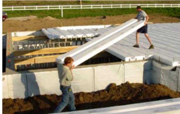
LiteDeck® sections are being placed on top of a solid, insulated concrete basement. The interior perimeter bracing and shoring (perpendicular to the clear span) has been placed. Note the vertical reinforcing steel which has been cast into the basement walls. That steel will be structurally integrated into reinforcing steel used for the LiteDeck® floor.
